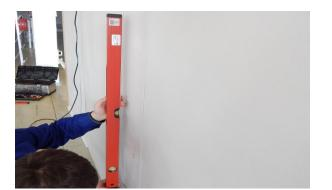
Check the vertical level of the cable. If necessary, correct by moving tightener in the bracket.
