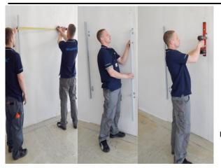
9. Use measure tape and spirit level to transfer installation places for second guide rail.
