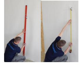
1. Designate spots in the axis of installation of brackets to the base. Put the bracket on the base and mark places for installation holes.
