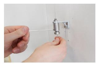
5. Put cable through façade tightener.
